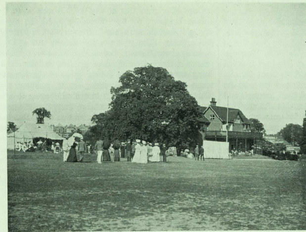
ATHLETIC GROUND, WINCHMORE HILL. THE PAVILION.
