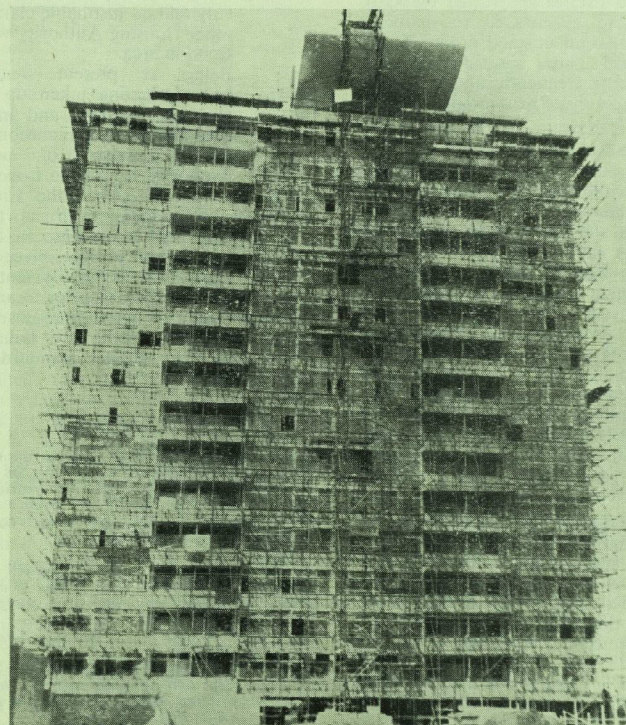
The Golden Lane Scheme: Flats in Construction.
