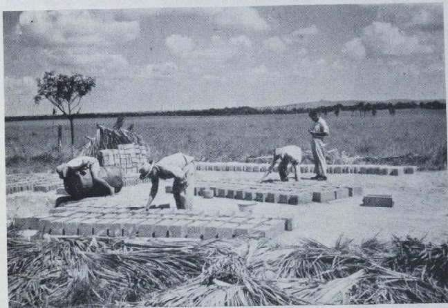
Adobe for haciendas. The ité fronds are used to control the rate of sun-drying of the puddled and moulded clay.
