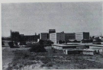
Hospital wards under construction at the All-India Institute of Medical Sciences.
