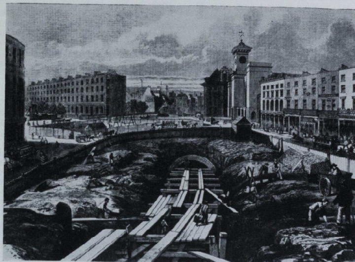
Construction of the line at King's Cross.
