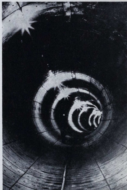
EXPERIMENTAL TUNNEL, CONSTRUCTION OF THE VICTORIA LINE
