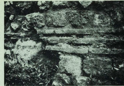
FIGURE 7. Wall. St. Alphages Gardens.
