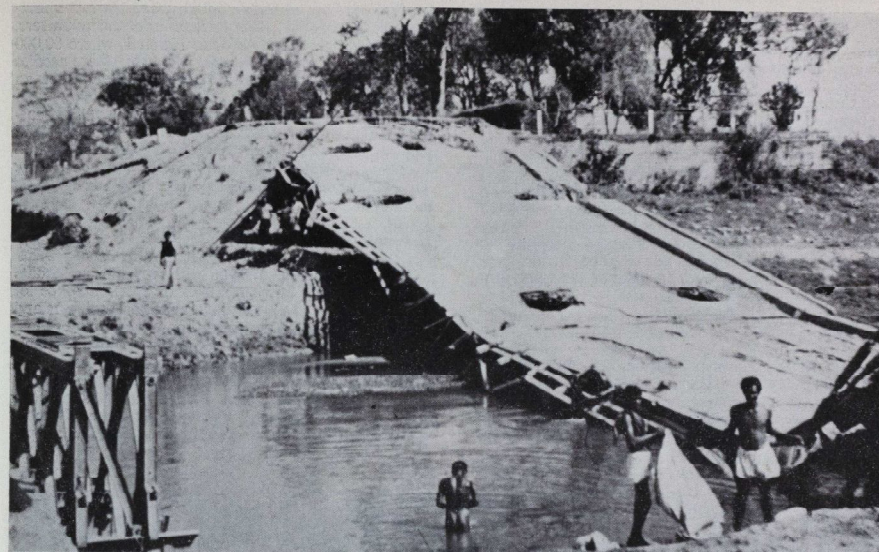
Bridge blown up.
