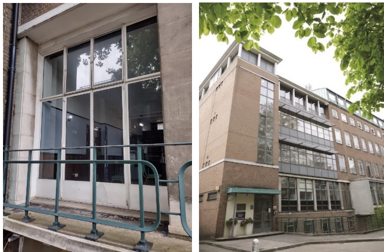
Figure 2: Examples of windows/doors in buildings of the Charterhouse Square Campus
