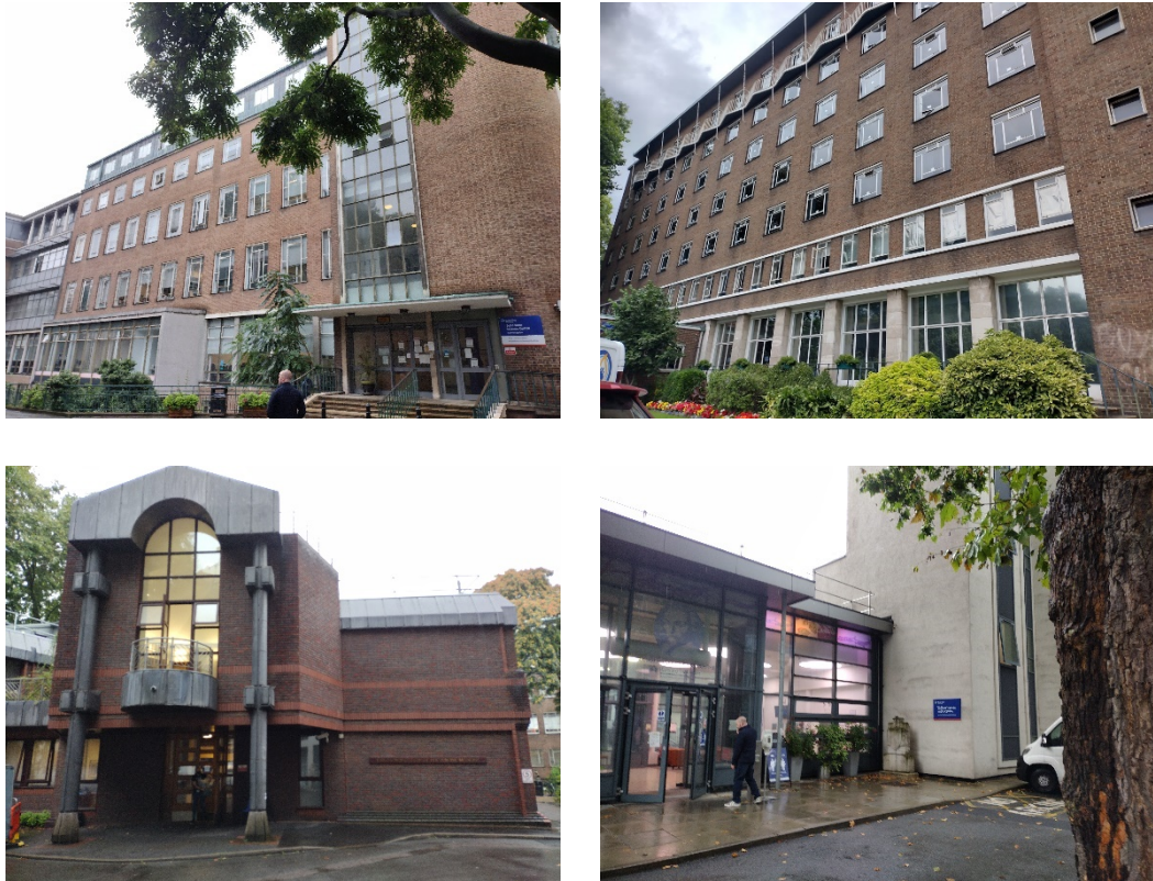
Figure 1: Examples of outside walls in buildings of the Charterhouse Square Campus
