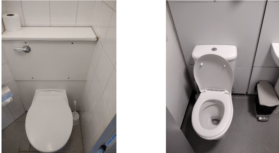
Figure 15: Examples of the one and two-stage toilet tanks
