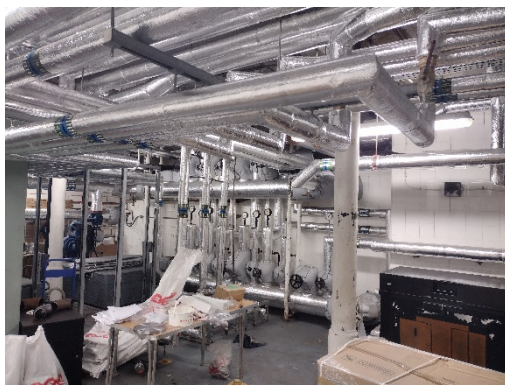
Figure 5: Examples of heating pipes insulation
