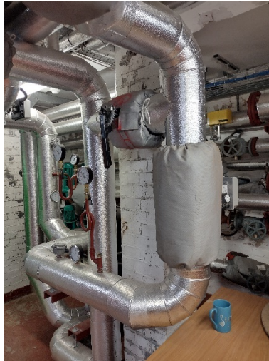
Figure 5: Examples of heating pipes insulation
