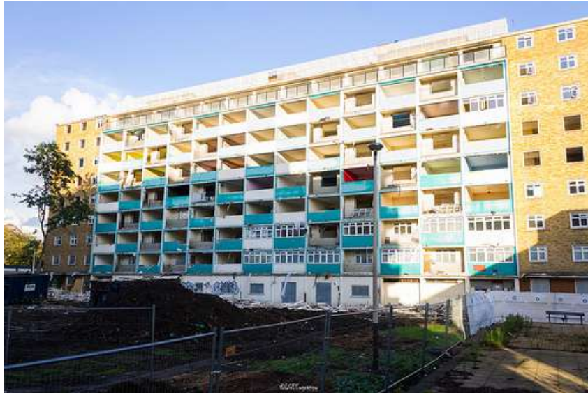
Panel A. Existing building
